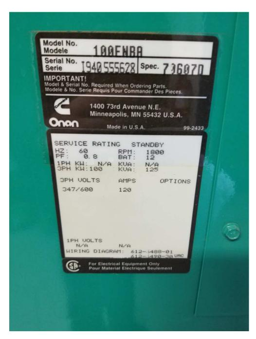
PHOTOGRAPH 10: McPhillips Regional Pumping Station – Collections Building - Generator Nameplate (all three generators are identical)
