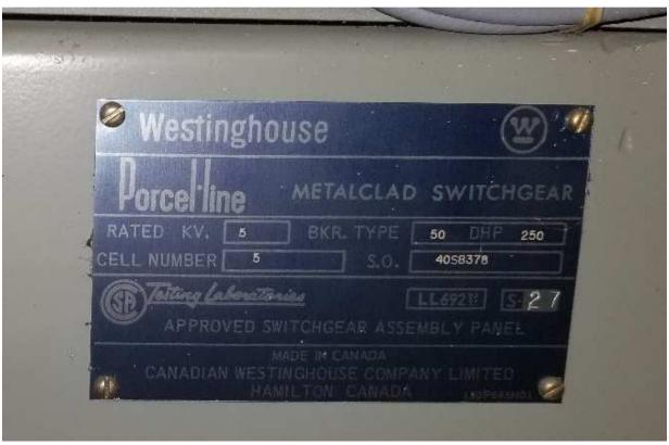
PHOTOGRAPH 5: McPhillips Regional Pumping Station – Main 4160V Switchgear SGR-M1 nameplate
